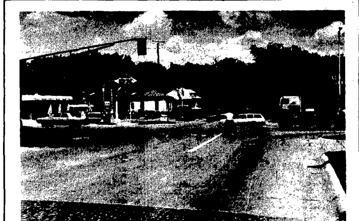
TRAFFIC CONFUSION at Seventh and Main will be cured, says the state roads department. Overhead signs will go up, new directional arrows will go down in a few days.
